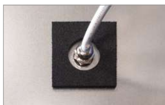
Waterproofing of the power cable
